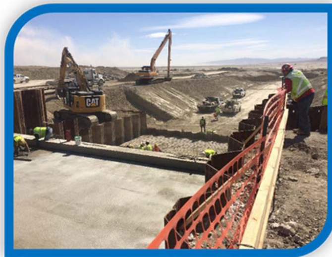
Photograph of construction during the 2017 “Big Dig” in Churchill County
