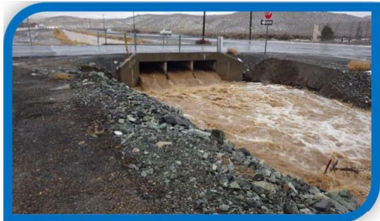
Culvert in Douglas County was upgraded to convey higher flow events
